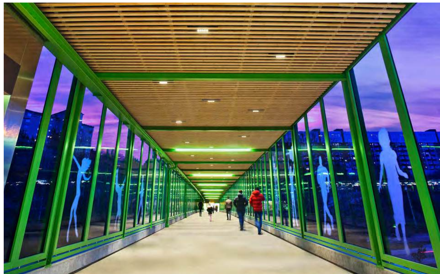
Project: Hallunda Station, Sweden
